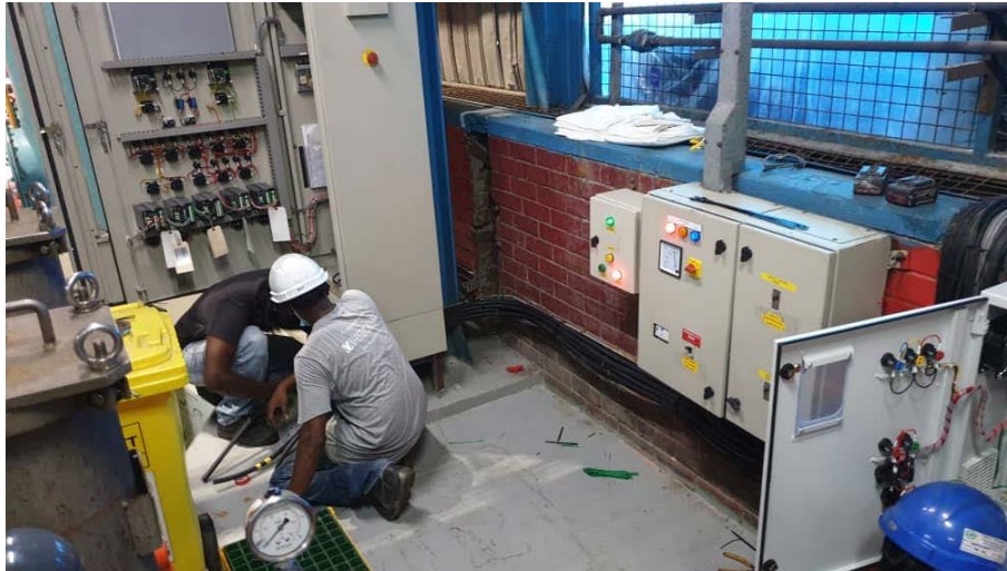
Inverter installation work - Bangi
